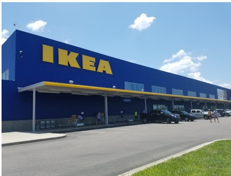
Figure #3: City of Tampa Brownfield Project.
